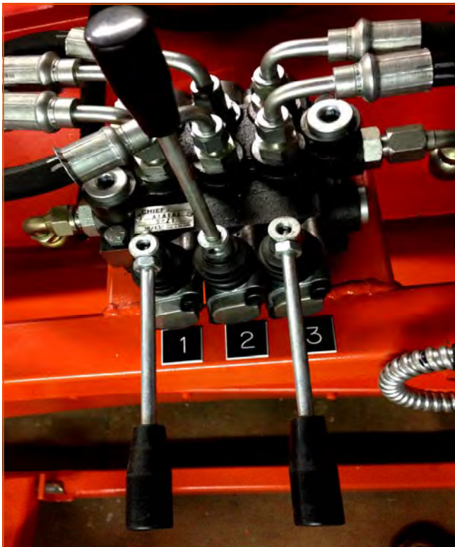
Control Manifold for Cylinders 1-3
